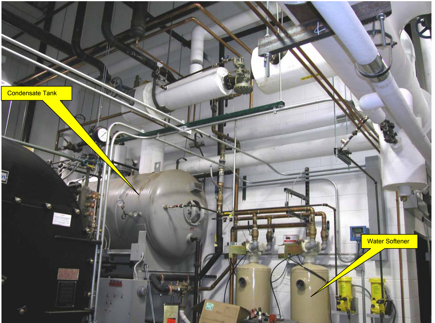
Figure 11 Condensate System
