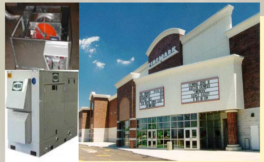
Theater: ICE/Desiccant Electric Load Reduction & Desiccant Dehumidification
