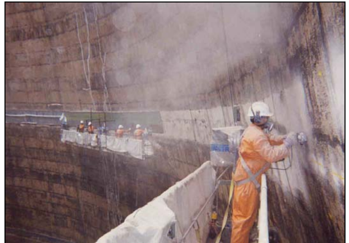
FRP Composite strengthening was applied inside the tower from cradles
