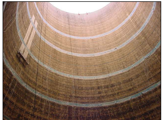
Strengthening bands within the cooling tower
